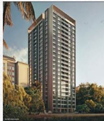
Rustomjee Reserve Mumbai 22 Storey High Rise Tower
