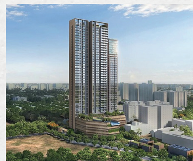
Tata 88 Kolkata 43 Storeys High Rise Tower
