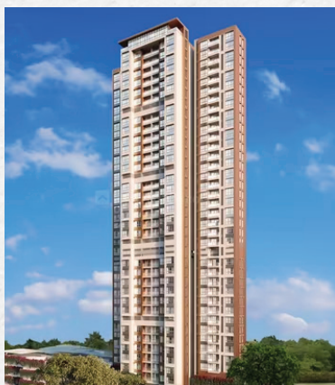
Piramal Revanta Mumbai 38 Storey High Rise Tower
